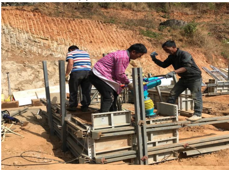
10/04/2019 夯牆培訓，開始夯牆
